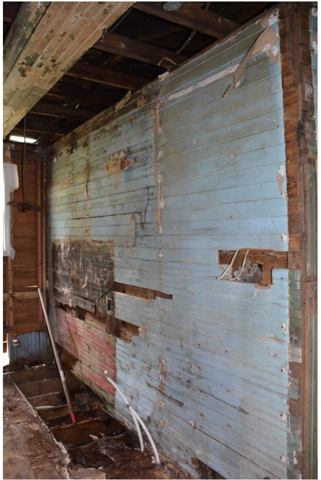
Kitchen, looking northeast, August 2015 (HF)
