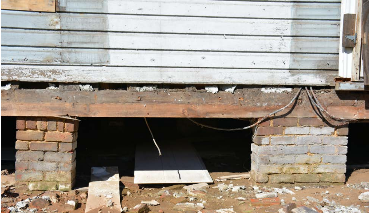
East elevation, foundation piers (HF)
