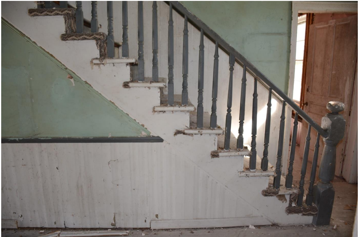
Center hall, stair, October 2015 (HF)
