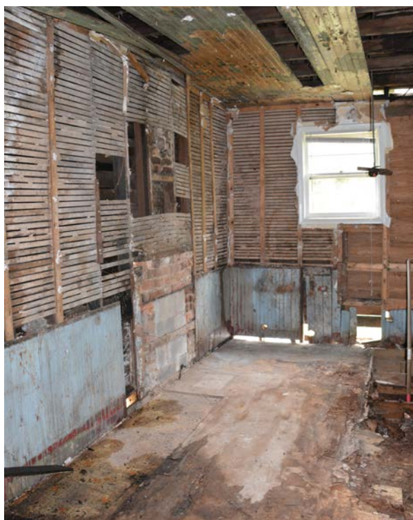
Rear addition, kitchen chimney (HF)
