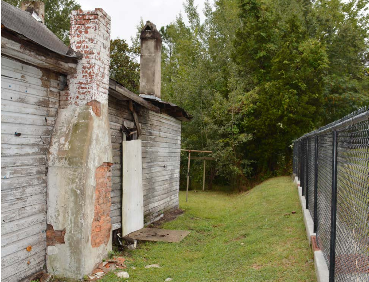
Rear addition, west elevation and cemetery fence, looking south (HF)
