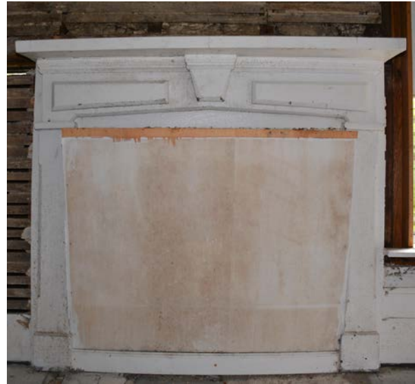
Second floor, north bedroom mantel (HF)
