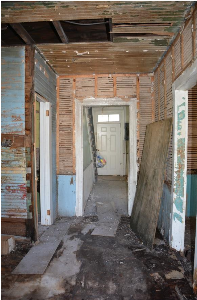
Kitchen, looking east, October 2015 (HF)
