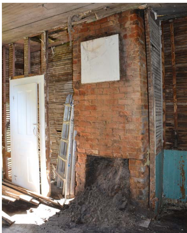
Rear addition, dining room chimney (HF)
