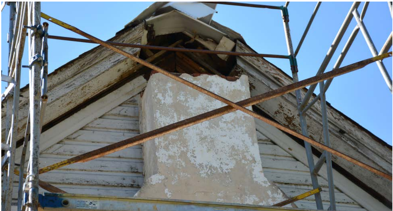
North chimney stack (HF)
