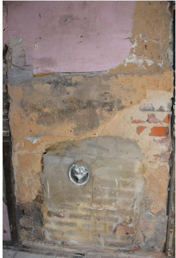
First-floor bedroom chimney (HF)
