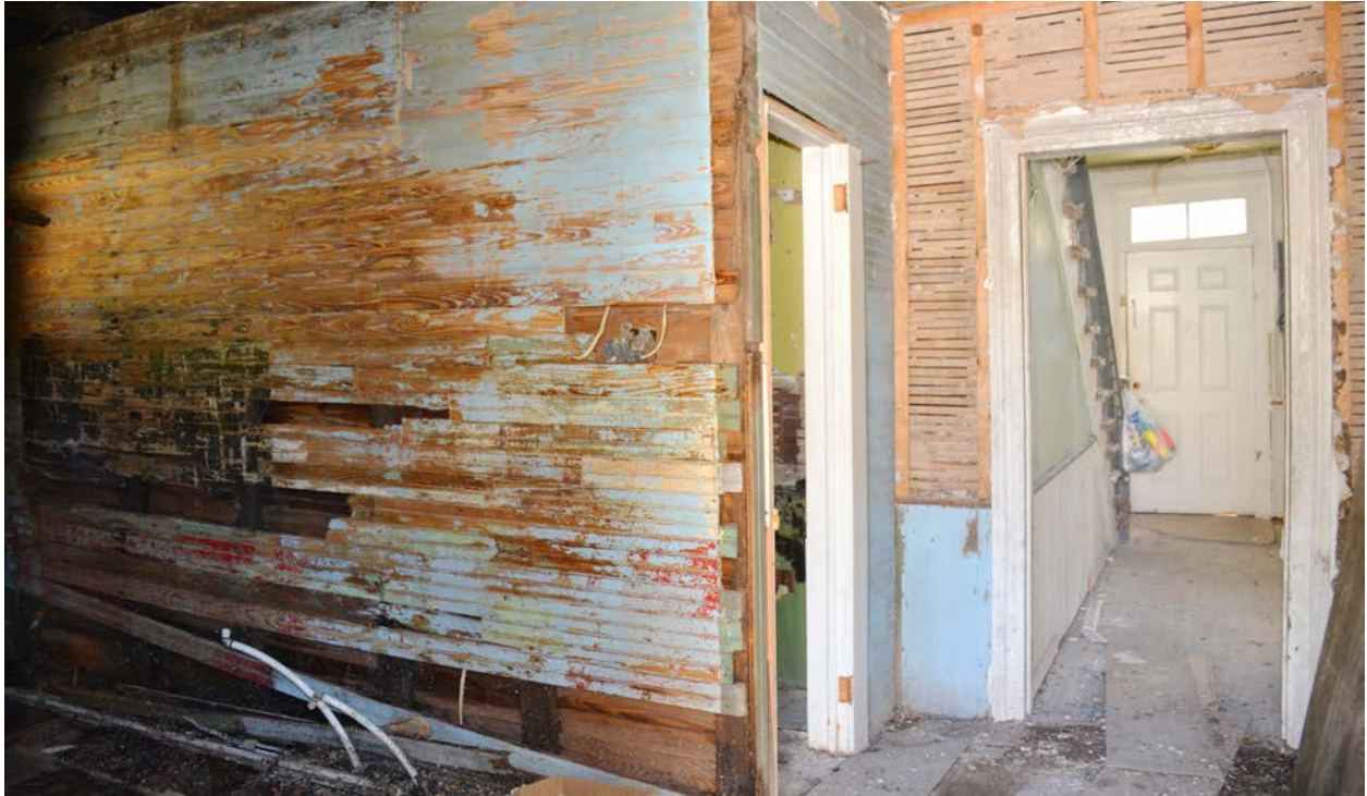
Rear addition, wall between kitchen and bathroom, looking northeast (HF)
