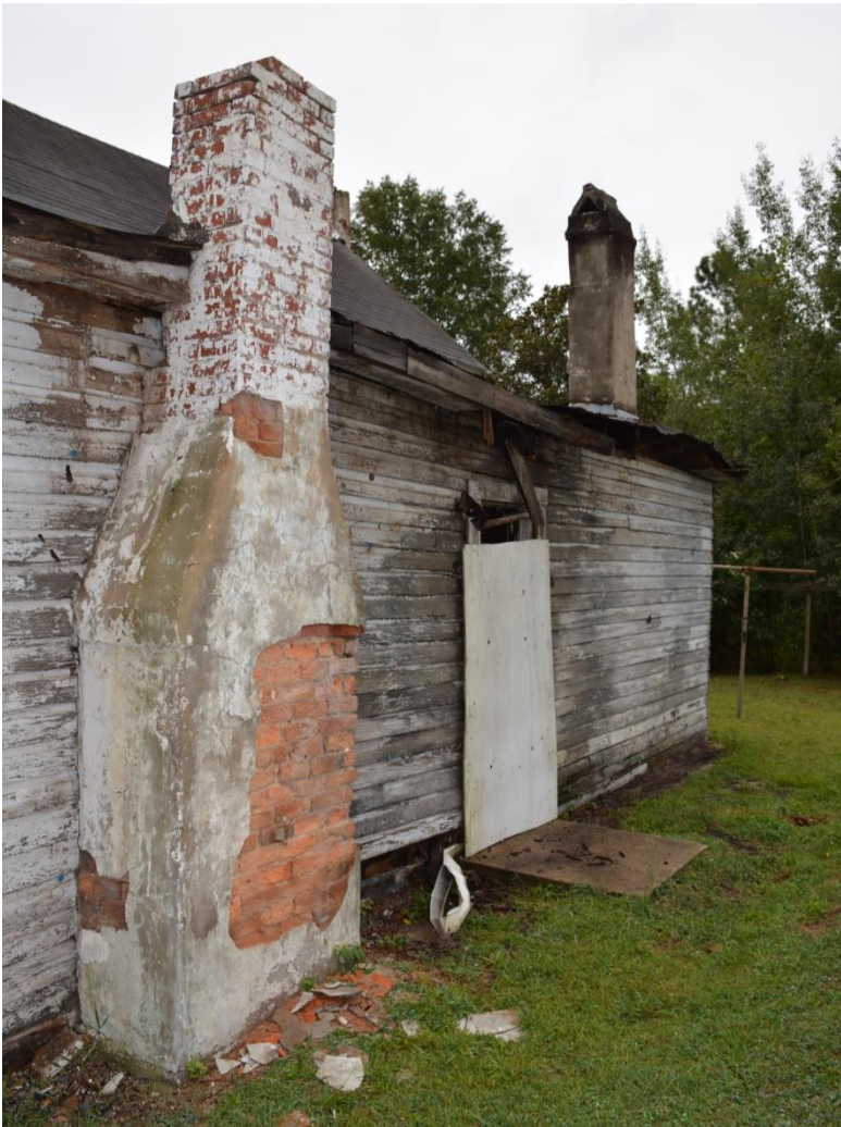
Rear addition, west elevation (left) and northwest oblique (below) August 2015 (HF)
