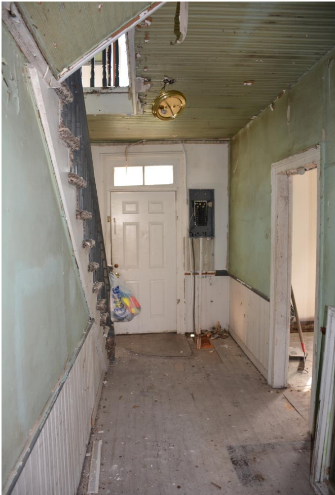
Center hall, looking east, October 2015 (HF)
