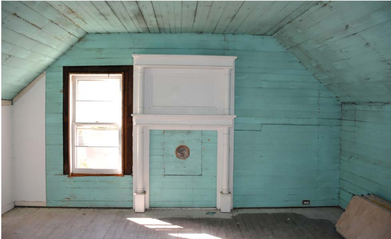
Second floor, south bedroom, looking south (HF)
