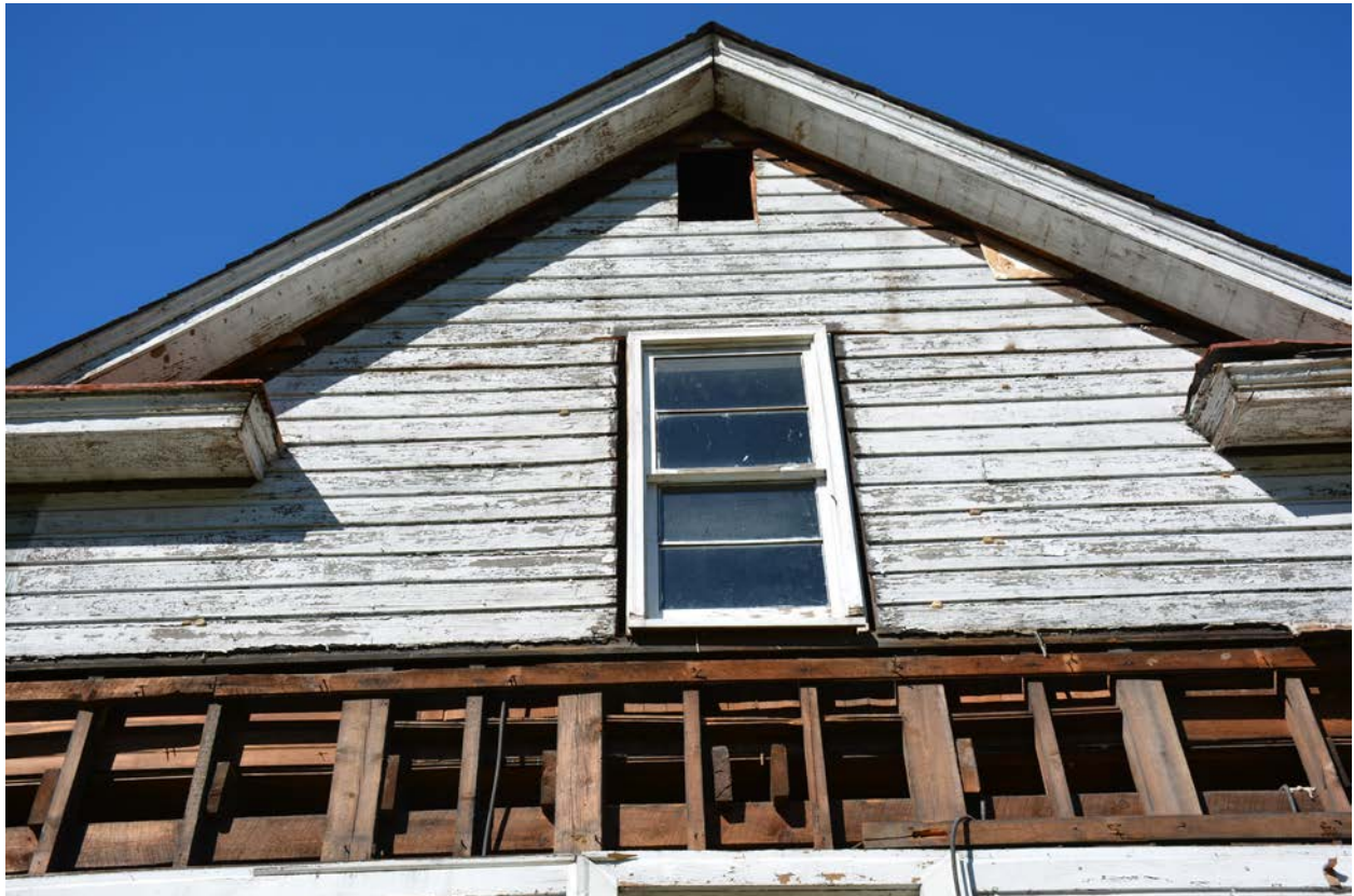
East elevation, front gable (HF)
