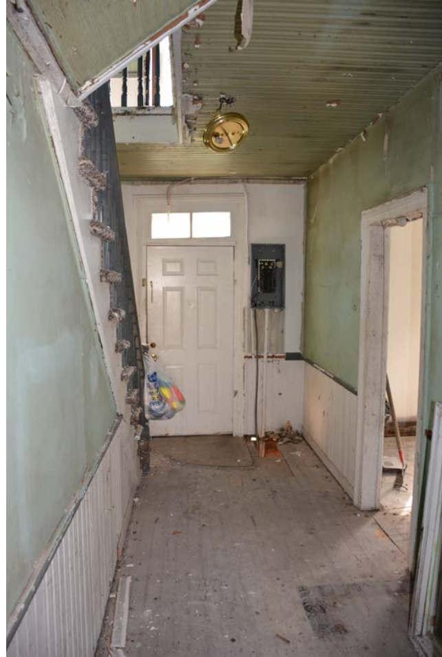
Center hall, looking east (HF)
