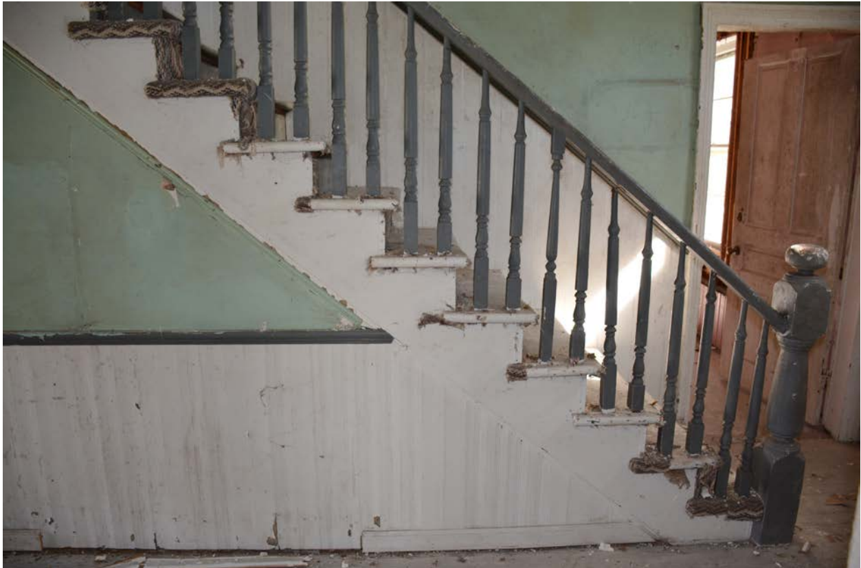
First floor, center hall, stair railing (HF)
